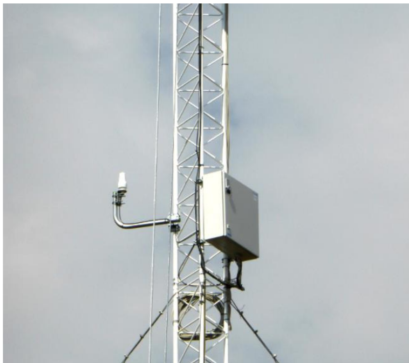
Fig. 66. Iridium antenna for satellite connection
