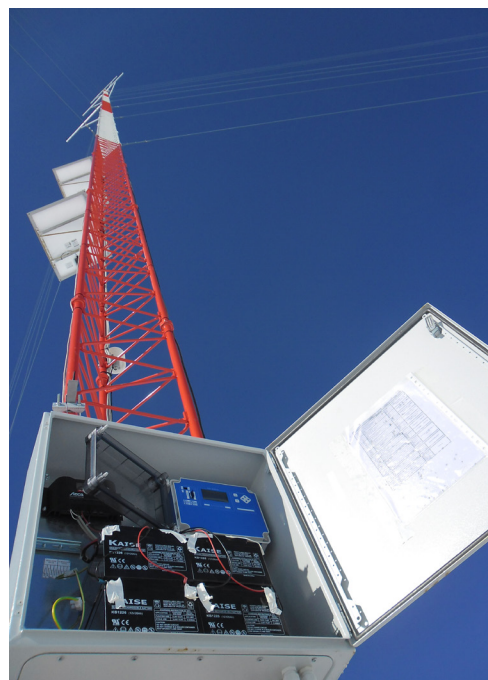
Metal cabinet prepared with data logger and battery backup.
