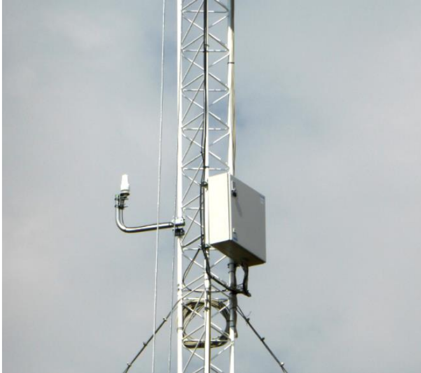
Fig. 61. Iridium antenna for satellite connection
